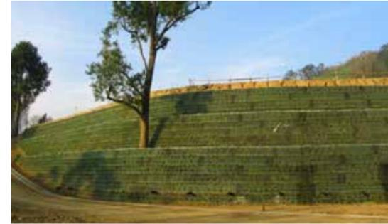
Based on the topography of the area, landscape planning and construction requirements, Wrapped Around Reinforced Earth Retaining Wall was constructed on the slope.
