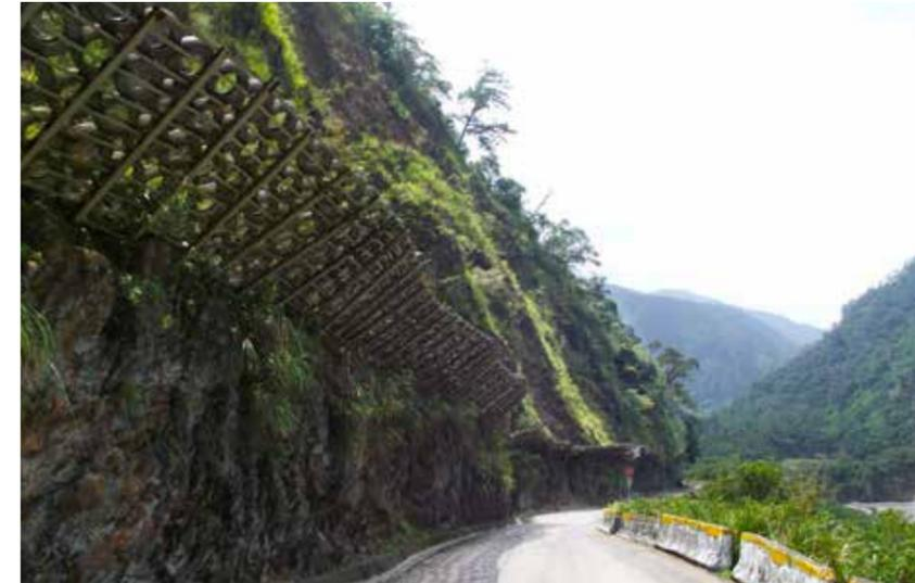
Self-drilling soil nails in combination with the anti-falling ACEMat™ R to stabilize the slope surface and the loosen/fractured soil layer to prevent falling rocks and improve the driving safety along the road.
