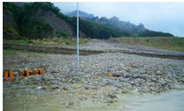
The schematic diagram in this section of rock-fall embankment prevention is shown below. Apart from the aforementioned energy dissipating function and earth retaining capability, another important aspect of earth embankment is that it can be constructed with debris material from the disaster and used as backfill material so that the local disposal cost and the working hours can be greatly reduced.
