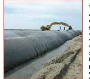
ACETube<sup>®</sup> Geotextile Tubes ACETube<sup>®</sup>, a large-sized tubular bag made of the polypropylene (PP) geotextiles, can be filled with sand and stones to form a gravity structure, which is usually used to construct various types of structures for shoreline protection. The bag material has good durability, good water permeability, sediment retention efficiency, and good workability, and as it can be filled with in-situ materials, it can also greatly reduce the construction cost.
