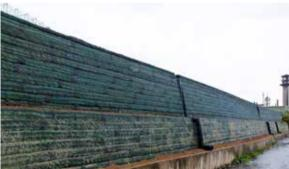
A 10m high-strength earth-retaining wall with a total length of more than 250m was built, and the top of the reinforced earth structure was used as a 15m-wide composite contact road.
