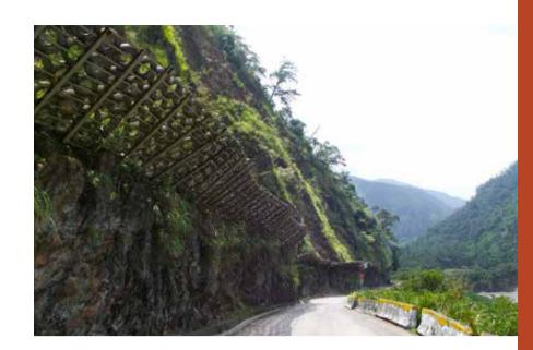
The three-dimensional ACEMat<sup>™</sup> R with diamond-shaped wire mesh composite was used to replace the traditional concrete slope which induces significant loading on the slope. Also, soil nail is used along the fractured zone to stabilize the slope surface, control the erosion of the collapsed ground and facilitate re-vegetation.
