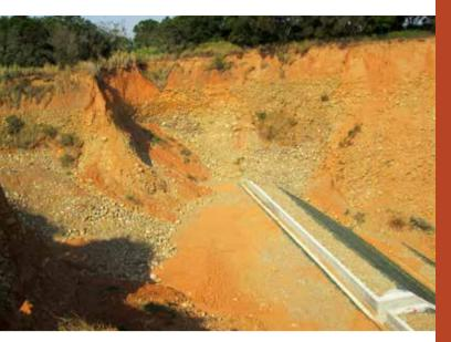
The mechanically stabilized earth construction method is used to complete the reinforced earth retaining wall at a height of 29 meters and the slope top drainage system.
