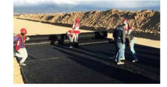
ACETex<sup>®</sup> geotextiles and ACEGrid<sup>®</sup> geogrids are used together, as the former separates the weak strata, while the latter reinforces and stabilizes the strata. ACETex<sup>®</sup> geotextiles and ACEGrid<sup>®</sup> geogrids can jointly disperse the building load and avoid soil subsidence to stabilize the strata.
