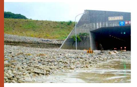
The stiffened earth embankment is used as the main structure for earth and stone treatment as it blocks and guides the earth and stones into the temporary accumulation area. A dredging channel is setup at the top of the embankment in order to transport and accumulate earth and rocks for reuse.
