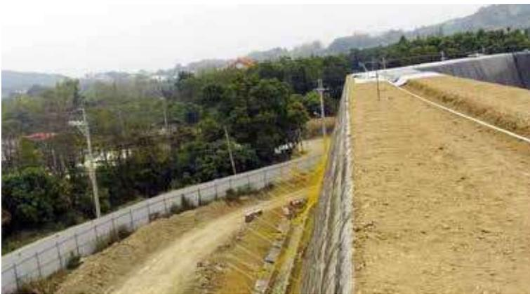
Over the years, population increase has reduced the capacity of Kaohsiung Class B Waste Landfill. Therefore, a facility expansion project was issued by the managing authority. Landfill construction was required to build a new containment system to accommodate future additional refuse. In order to reach a maximum capacity of the landfill, the perimeter dike slope must be built as steep as possible.
