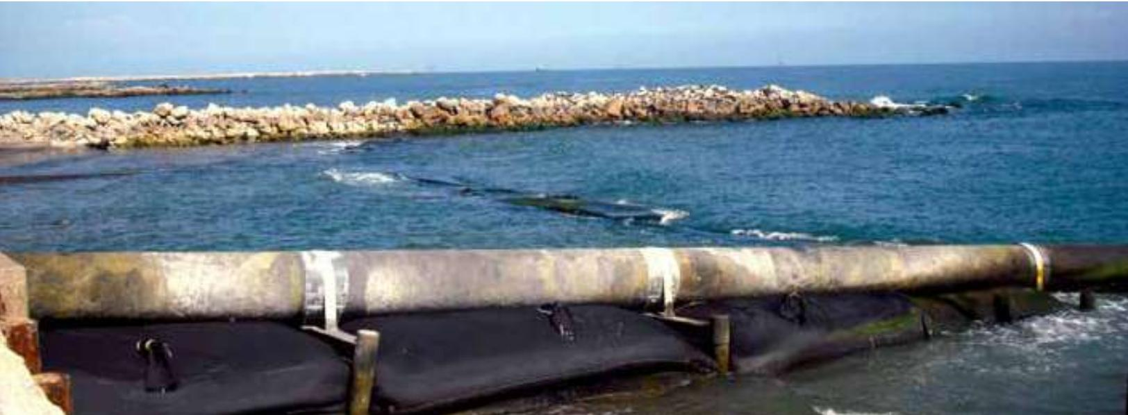
The marine facilities of Dos Bocas PEMEX, a major oil corporation in Tabasco, Mexico, suffered progressive beach erosion caused by numerous annual hurricanes invasion. The sand foundation under the pipelines in the littoral zone was scoured, leaving dangling pipes. Such problem threatened oil conveying and the integrity of the infrastructures. It also increased the potential risks of pipeline failures which would lead to economic loss and environmental contamination.
