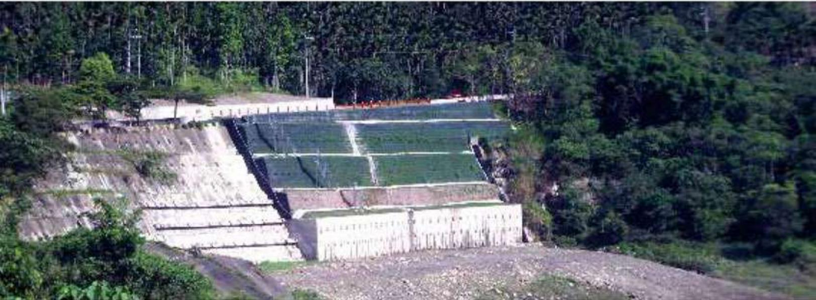
In 2007, torrential rainstorm caused a landslide with 80 m wide and 30 m deep in the fault zone of Nantou County. The existing anchored slope experienced a structural collapse, leaving a massive soil debris at the toe of the slope. Moreover, the site is located at the edge of Ming-Tan Reservoir, making it vulnerable to erosion due to the water level fluctuation.
