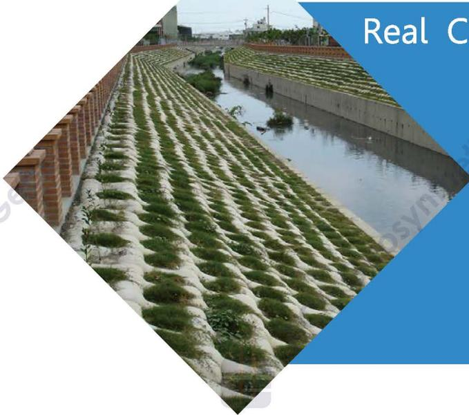
ACEFormer™ is applied in a channel broadening project as bank protection at both sides of the channel. The main purpose is to prevent the channel from erosion. The application of ACEFormer™ not only reduces the flow velocity of water, but also enables vegetation growth along the channel for a more pleasant appearance than cement finishing. The easy and rapid installation of ACEFormer™ helps the project to complete within schedule with high effectiveness.
