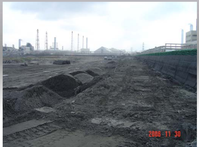
Construction of embankment
