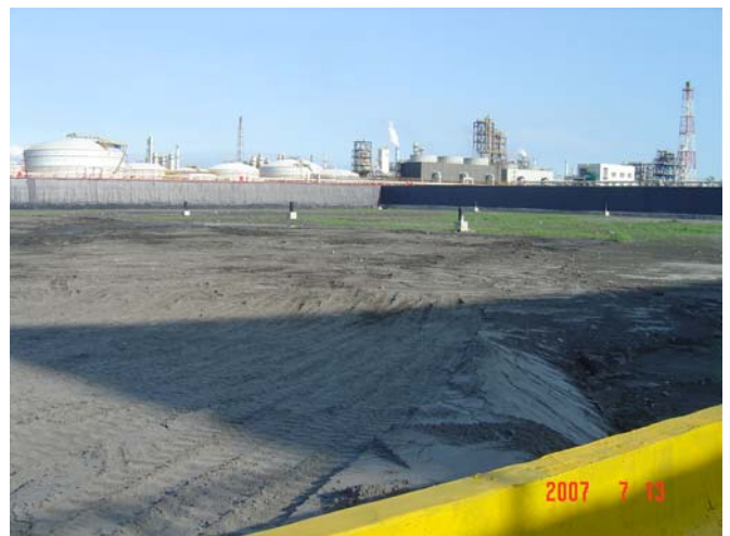
Construction of geomembrane
