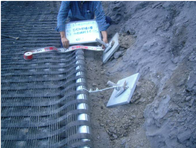
Figure 4. During construction (connection system)
