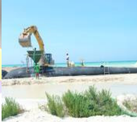
Filling ACETube® with Hopper
